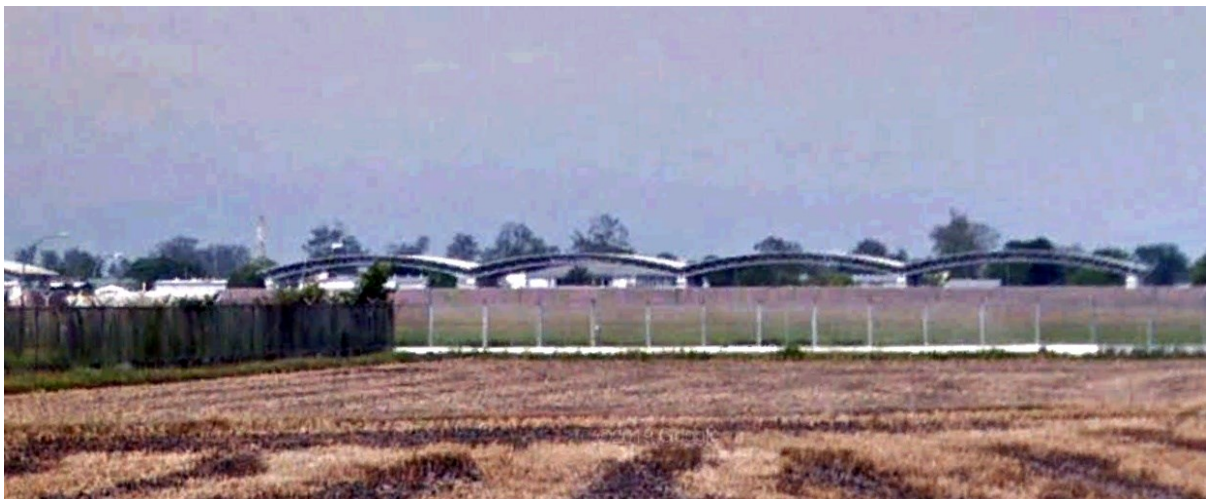
Figure 19 Butterworth hangars South West of the BW radar (Streetview)
